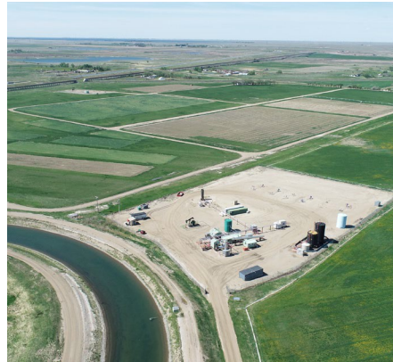
»» Bantry 15-23 Oil Battery and Sunburst Well Pad
