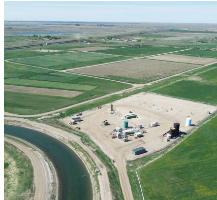
Bantry 15-23 Oil Battery and Sunburst Well Pad
