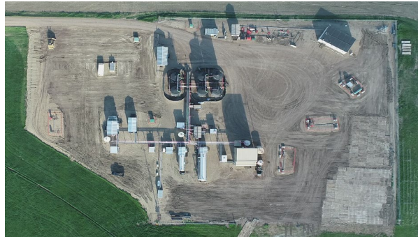
Overhead drone shot of the Bantry 2-29 oil battery
