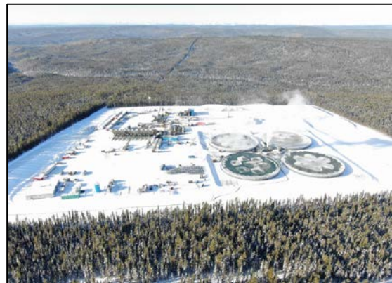
Figure One – Calima pad site during drilling operations
