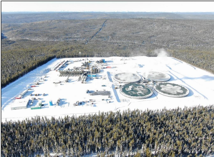
Calima pad site during drilling operations
